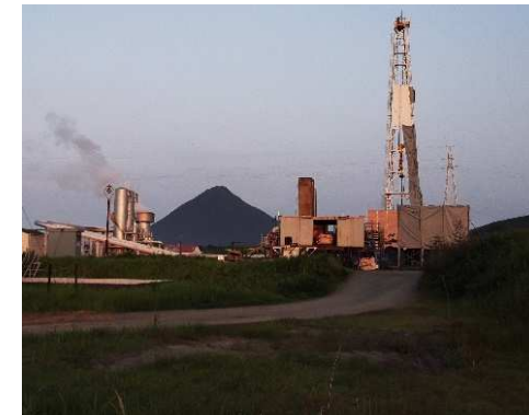
Geothermal power generation drilling site
