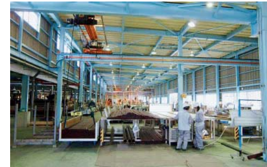
Tochigi Piping Plant
